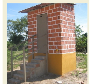
The new ecological composting latrines resolve issues of waste contamination related to health and the environment, as well as providing privacy.
